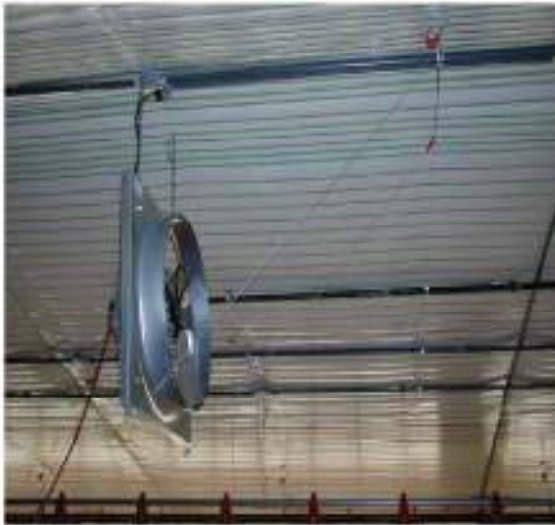
Low Ceiling House with 24-inch Panel Fans Installed. In these photos note the winching arrangement so that the fan may be pulled up out of the way during clean-out and catch.
