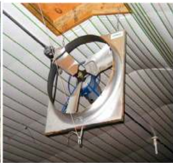
Low Ceiling House with 24-inch Panel Fans Installed. In these photos note the winching arrangement so that the fan may be pulled up out of the way during clean-out and catch.
