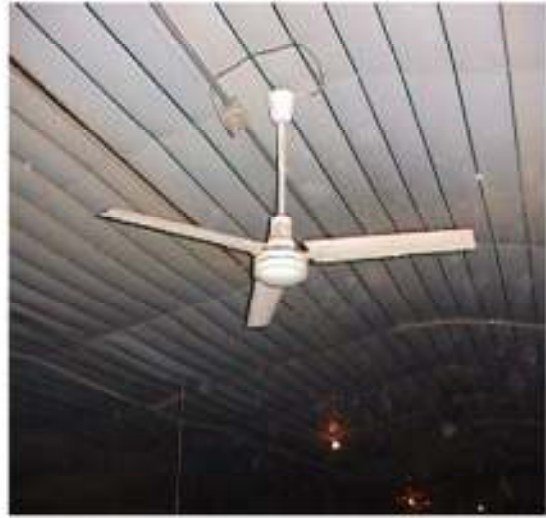
Low Ceiling House with Paddle Fans Installed. On photo at right notice cord and plug connection so that fan may be removed during clean out.
