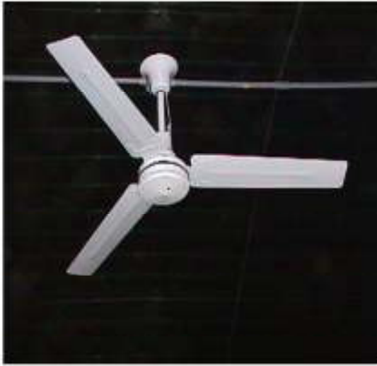
Low Ceiling House with Paddle Fans Installed. On photo at right notice cord and plug connection so that fan may be removed during clean out.
